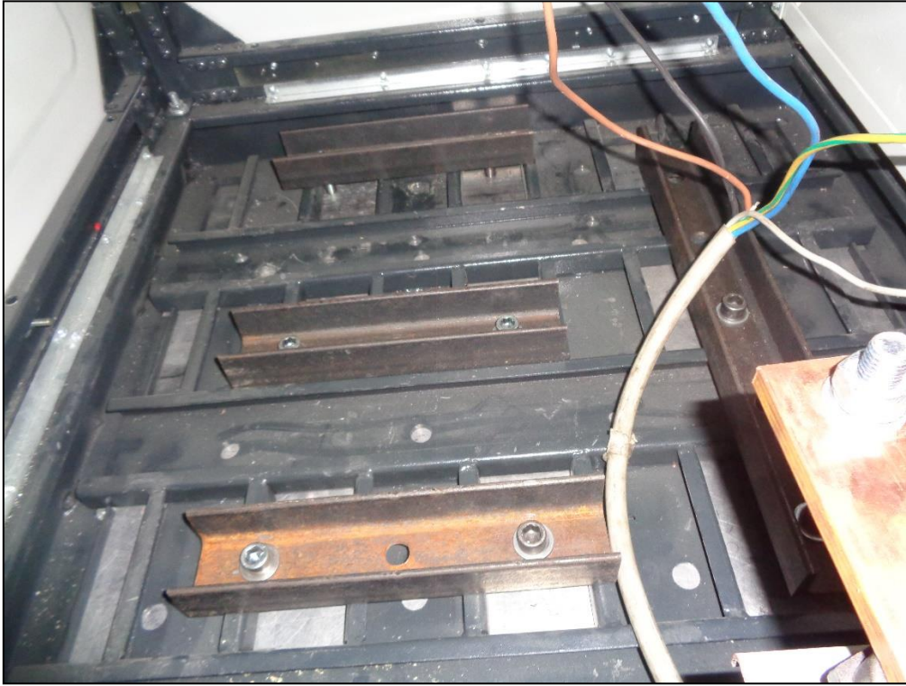
Photo 6 – Mounting technique – Power cabling
